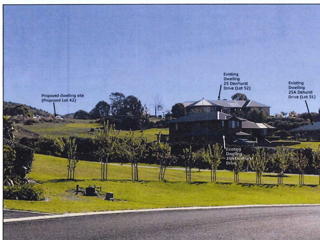
Plate 1: View of the subject land to North West from Dewhurst Drive
