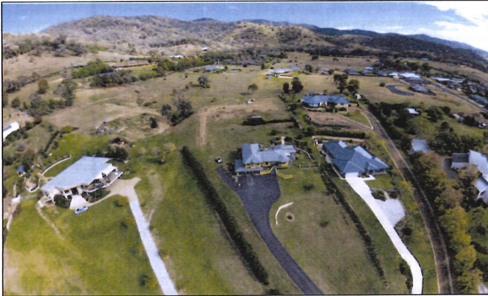
Plate 5: View of site depicting level building opportunity adjacent existing dwelling (May 2016)
