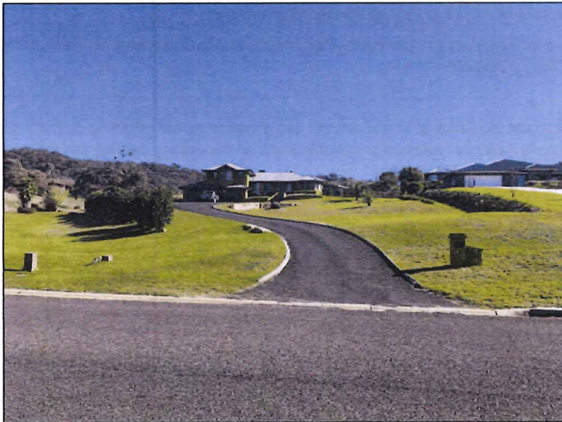
Plate 2: View of 25B Dewhurst Drive from frontage to Dewhurst Drive
